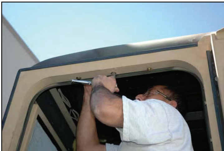
3.) Tighten bolts on frame of door.
